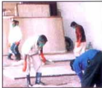
Prorer use of PPEs - Mask Prorer use of PPEs - Hand Gloves Prorer use of PPEs - Rubber Boots
